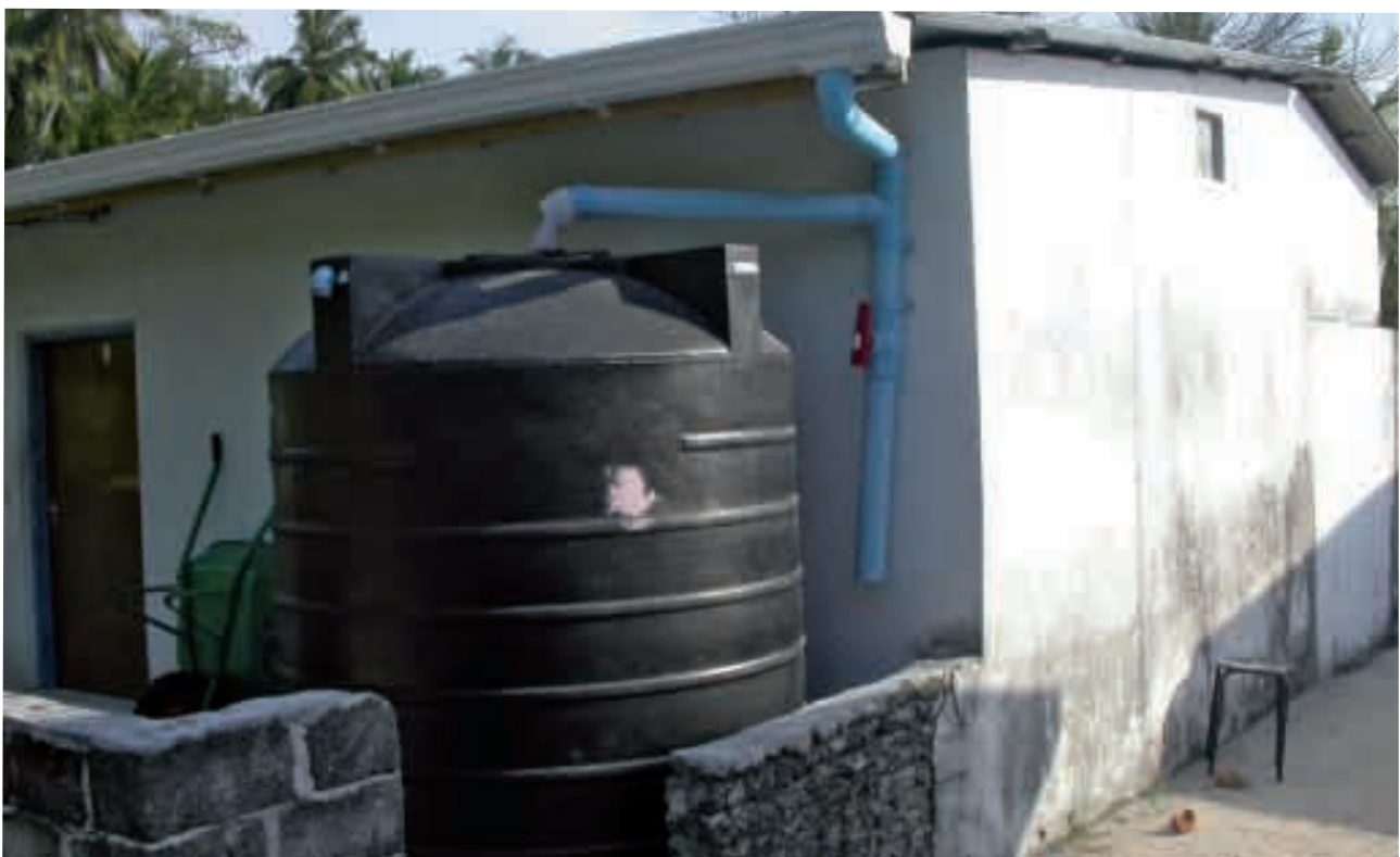
Water storage containers-Are they safe?
