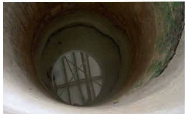
The well should be cleaned regularly!
